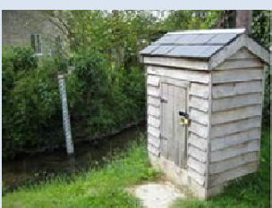
The Environment Agency installed a flood monitoring station on the River Churn as a result the parish plan
